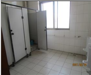
Photo of the sanitary facilities Toilet.JPG
